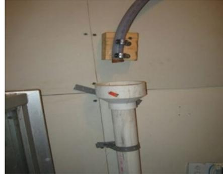
*Softener discharge drain line with air gap*
