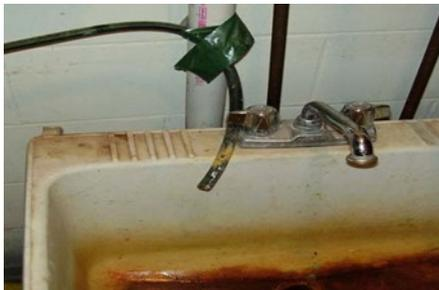
*Placing the softener discharge drain line into a sink without an air gap*
