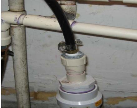
*Softener discharge drain line directly plumbed to a sewer*
